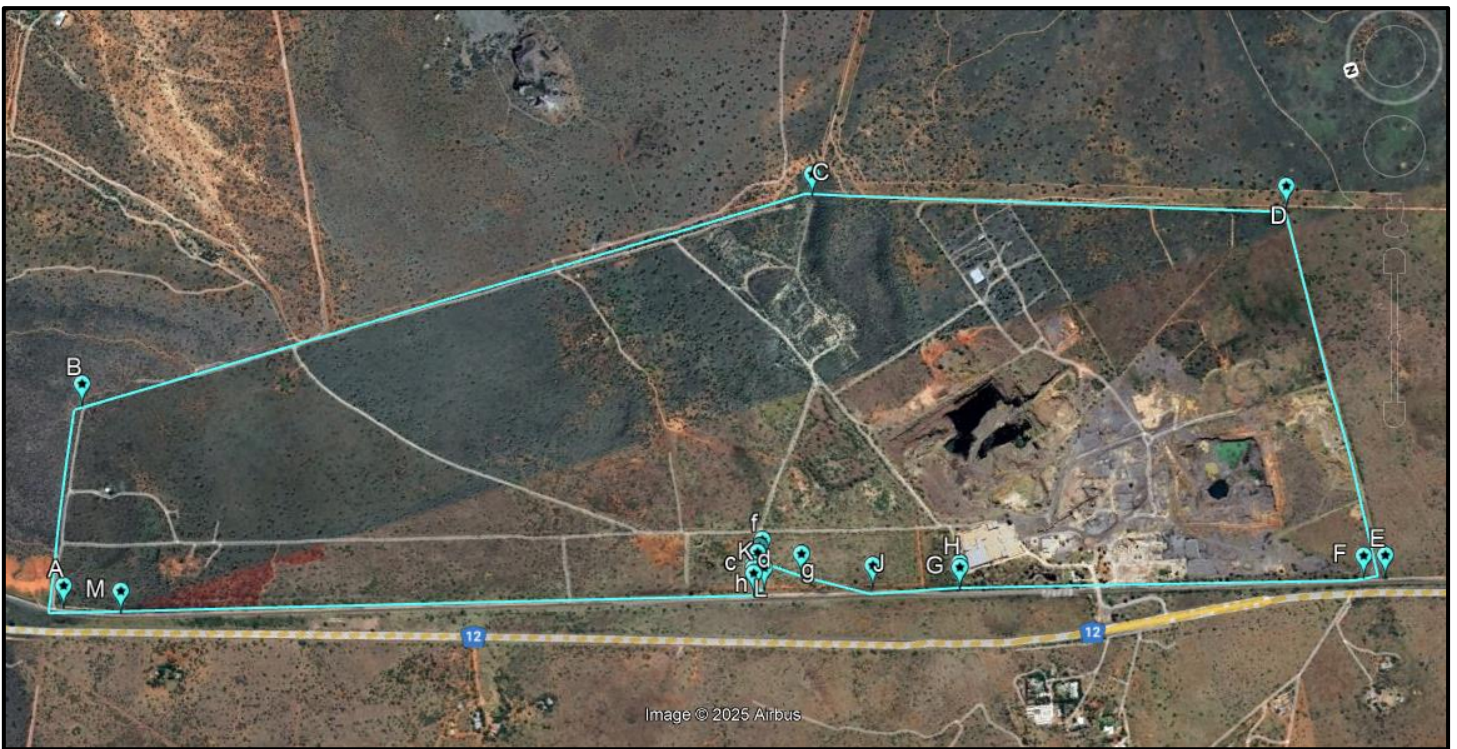
Figure 1: Satellite view of the Kimberley Quarry mining footprint (image obtained from Google Earth). Note: To optimise space, true north is directed to the left.
